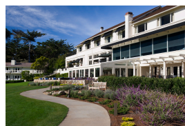
The Bench Restaurant renovated in The Lodge at Pebble Beach, Calif.
