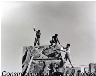
Construction continues at Taliesin West, with apprentice Arnold Roy on right, 1956. Courtesy A. Roy.
